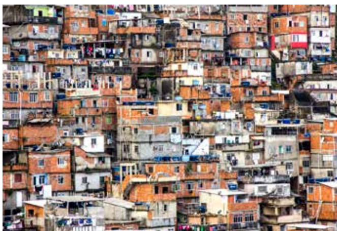
Figure 11: In the heart of a highly built-up and paved area of a Rio de Janeiro favela, with extremely hot temperatures all year round, green roofs can make a big difference.
