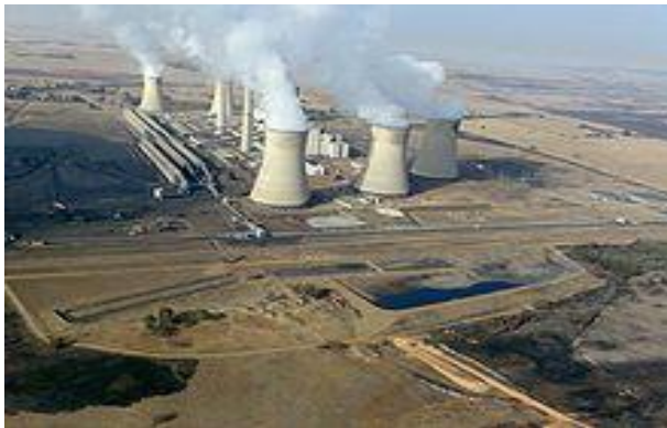
Fig.4.18 The Anort Power Station in Mpumalanga
