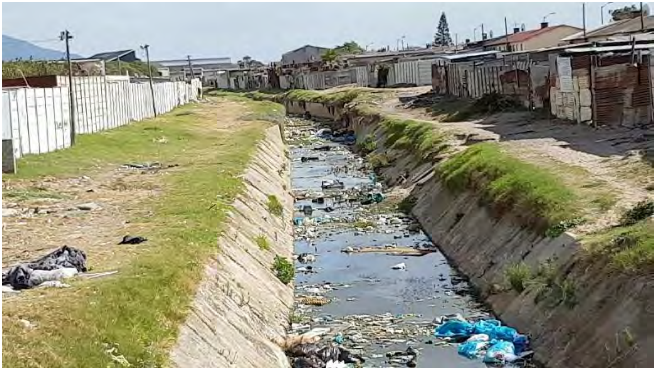
Figure 6-12 Section of the Lotus Canal as an example of the pollution and degradation of a previously natural stormwater run-off system (Hay, 2019)
