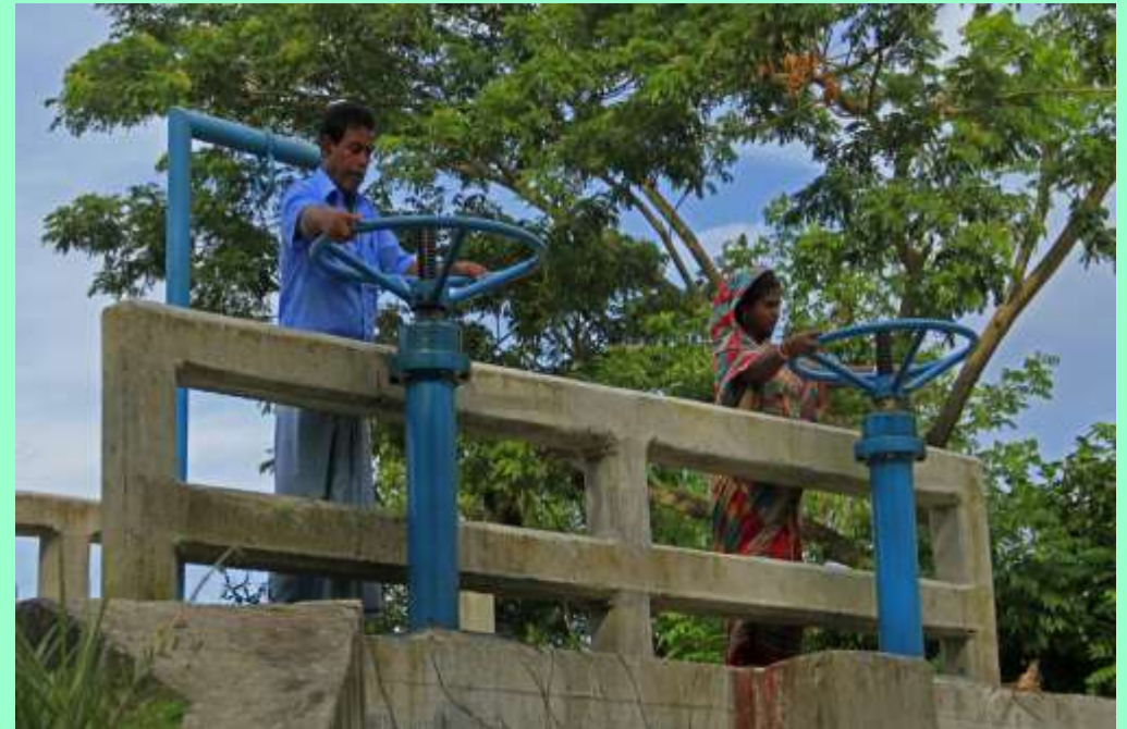
Members of a Water Management Group operating a sluice gate in Bangladesh (Credit – Blue Gold Program, Bangladesh)
