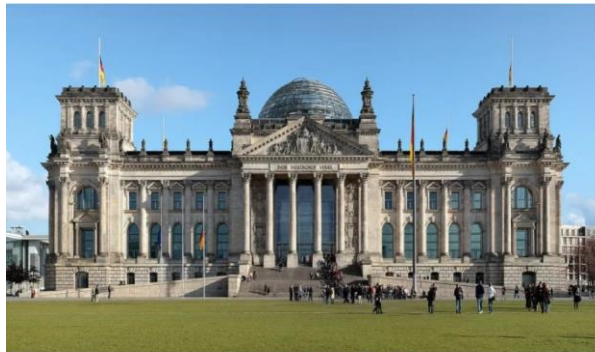
Western side of the Reichstag building, Germany's parliament lower House in Berlin. Photo credit: Matthew Ford
