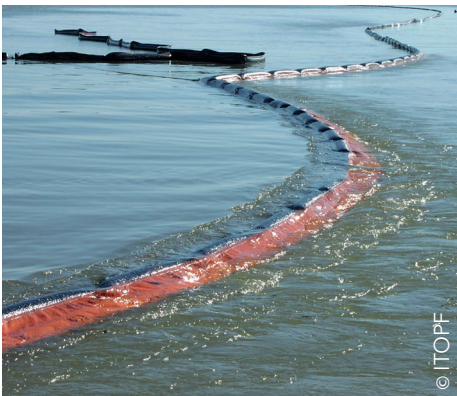
Boom failure due to strong currents
