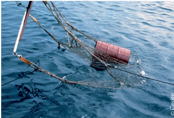
Lifting a drum with a collection net
