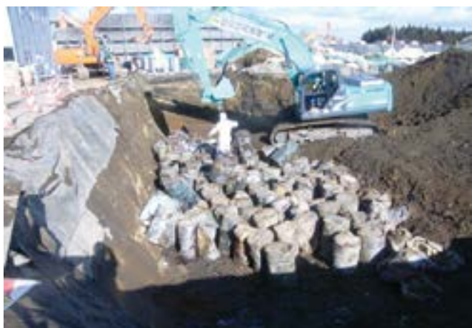
Figure 1. Removal of illegally dumped waste (Source: Iwate prefecture)
