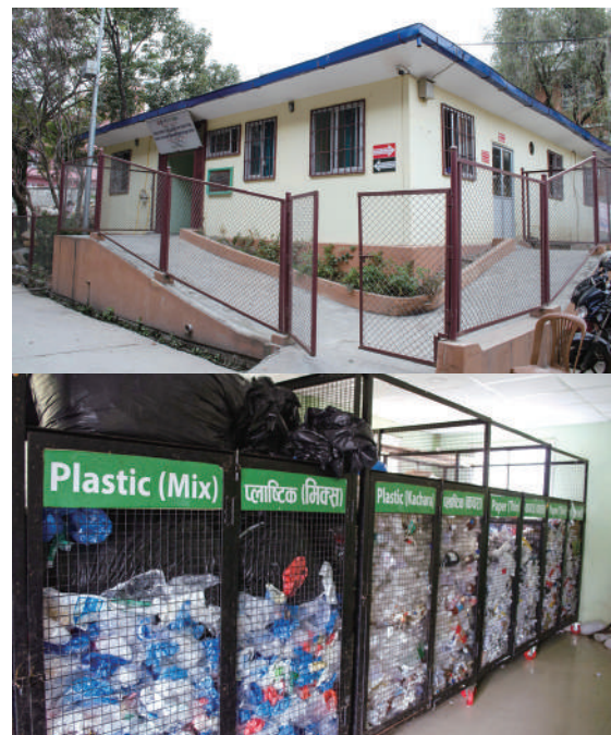
Figure 13: The waste treatment centre (top) and Storage for recyclable wastes (bottom) (Source: HECAF 360)
