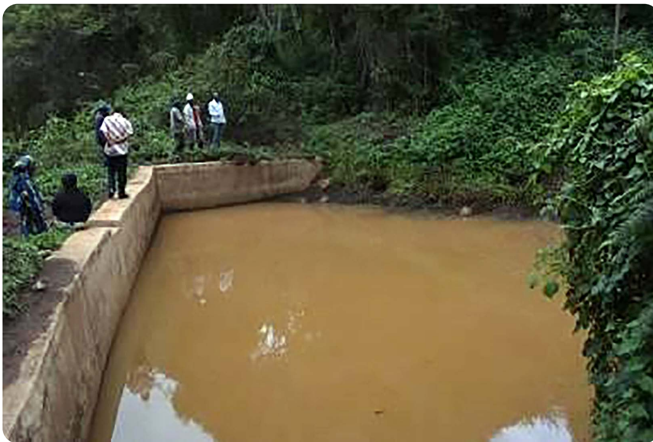
Constructed ndiva supported with concrete ©Hans Komakech
