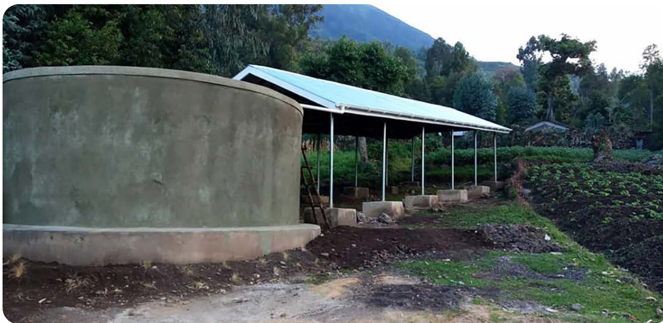
A water tank in Kabande village ©Water for Virungas (W4V)
