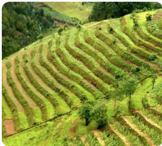
Terraces built on a steep slope ©FONERWA
