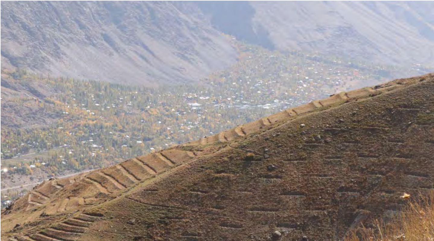
A series of terraces and stone bunds on the slopes of Deh-shahr catchment
