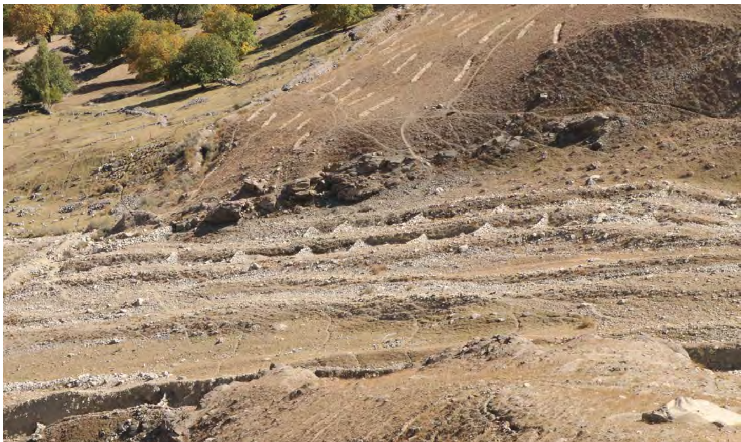
Check-dams, soil bunds and tree plantations help stabilize slopes
