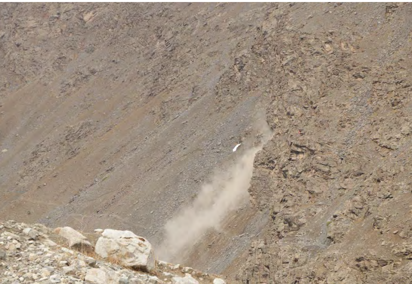
Cutting through hard rock during Oshtuk canal rehabilitation
