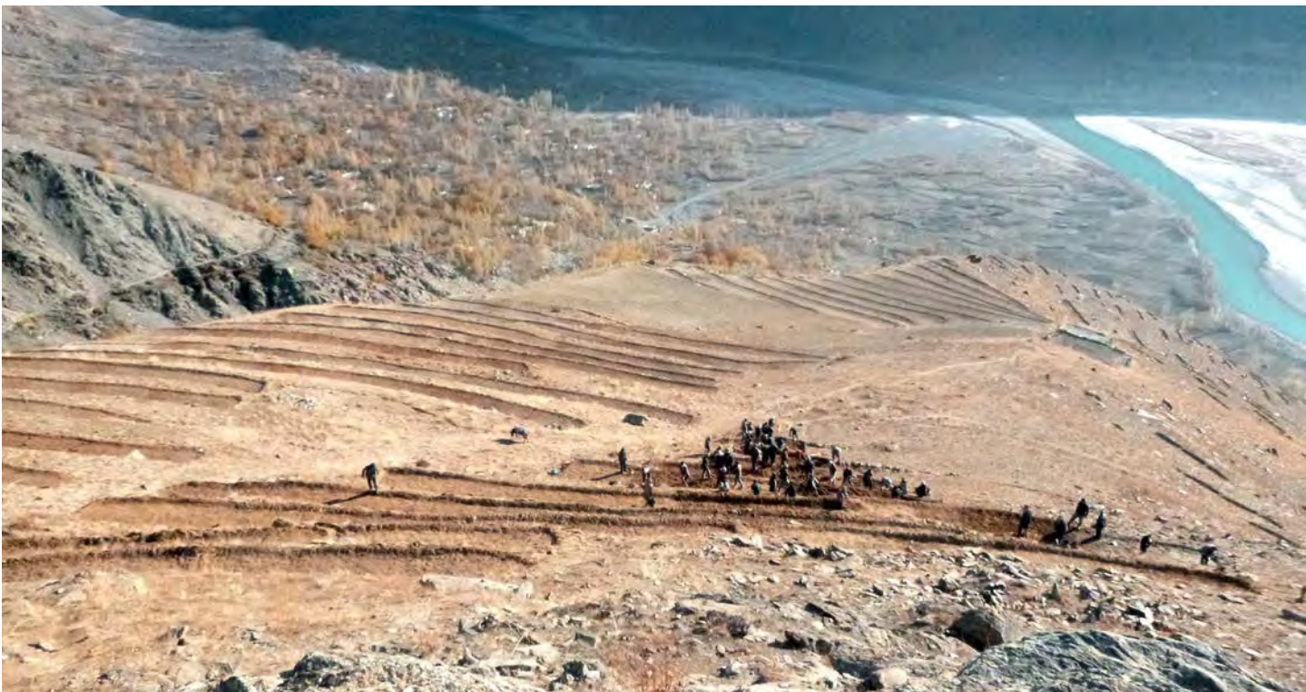
Community members constructing terraces
