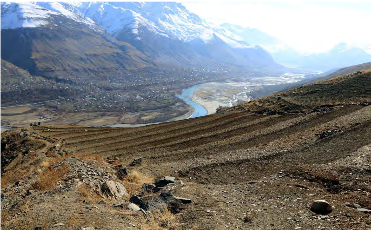
Terraces were constructed to stabilize slopes and limit soil erosion
