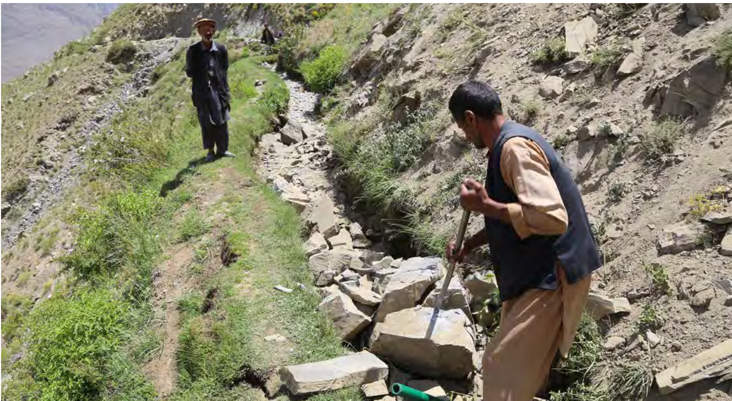
Rehabilitation of mountain irrigation canal using dry stone building technique
