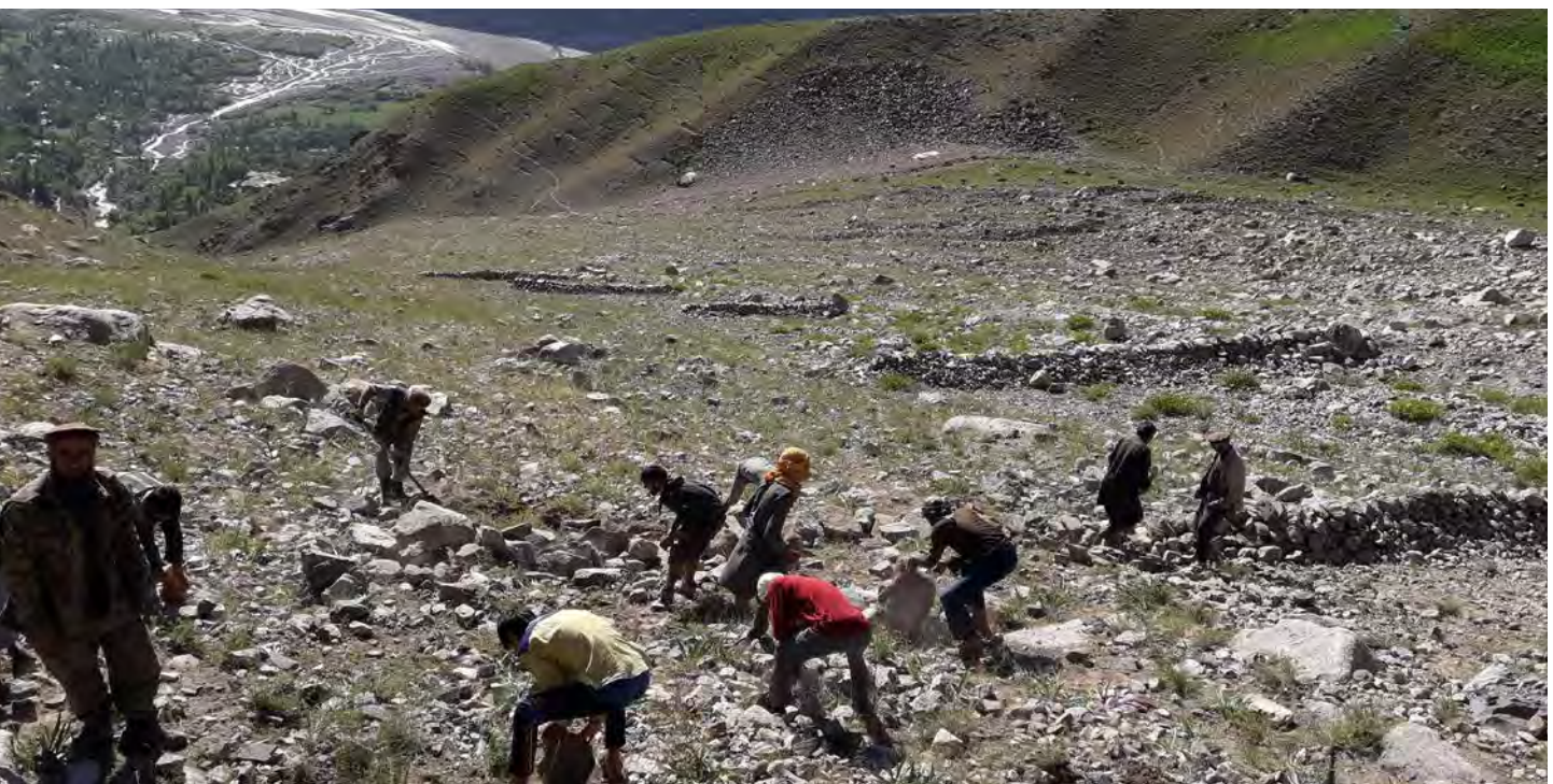
Construction of gully plugs or check-dams in the upper catchment area
