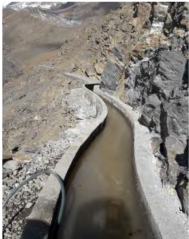
The completed canal in a rocky outcrop segment
