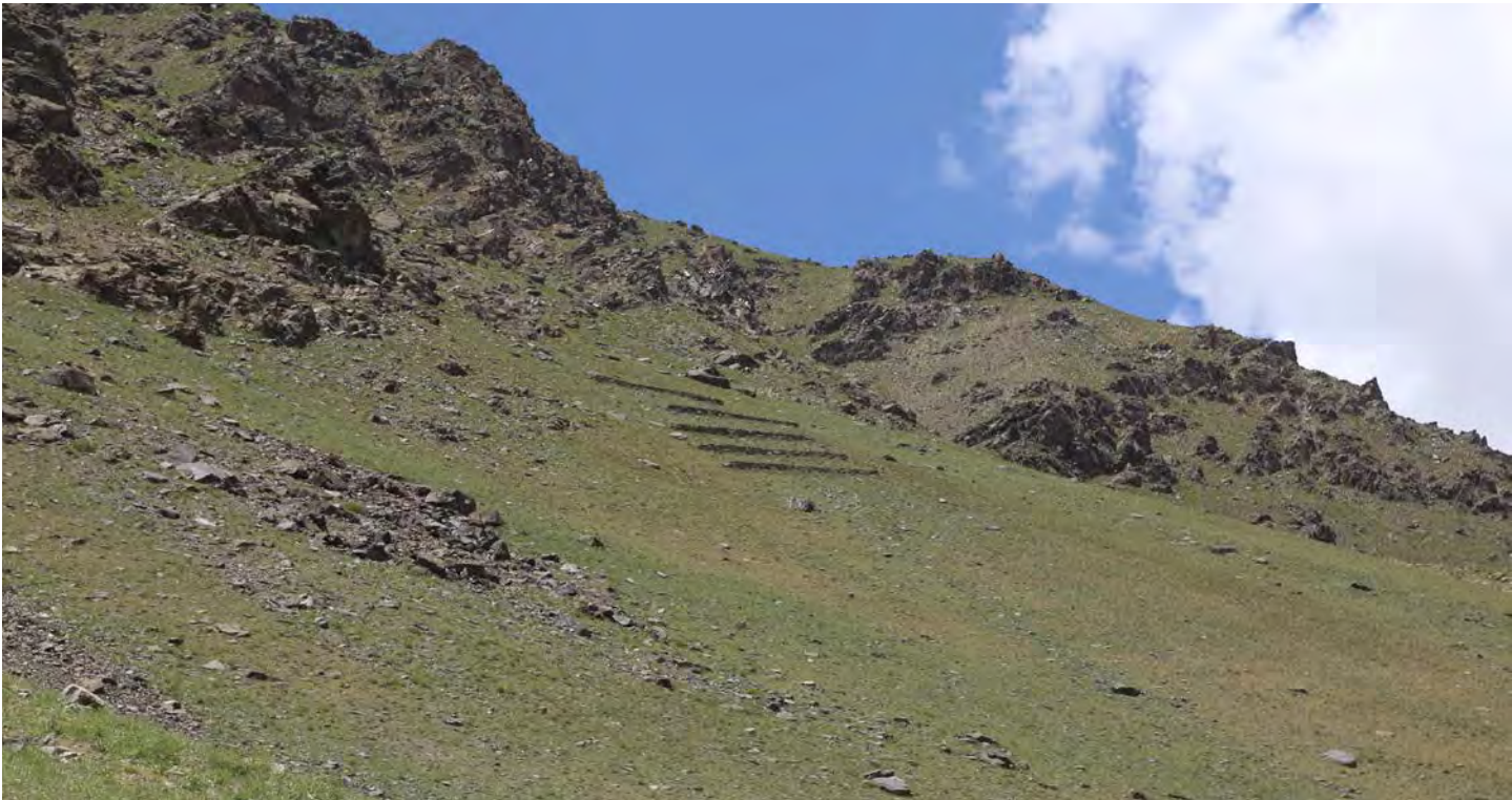
Avalanche prevention structures
