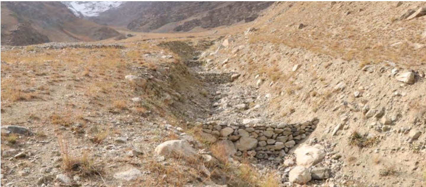
Gully-plugs reduce the risk of flash floods and avalanches
