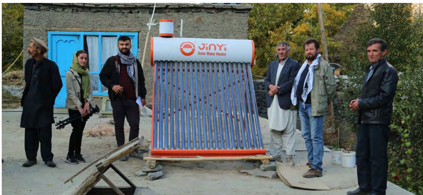
Solar water heaters were installed in 125 households
