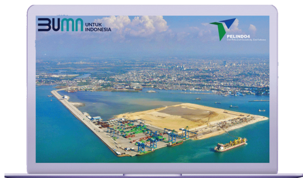
Figure 30: Makassar New Port development
