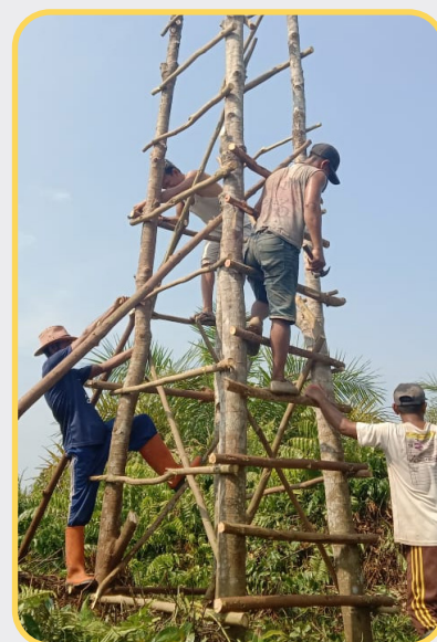
Community groups voluntarily build the peat fire monitoring tower using their own resource. Photo Credit: Vernando Maruli Aruan/ Wetlands International Indonesia.
