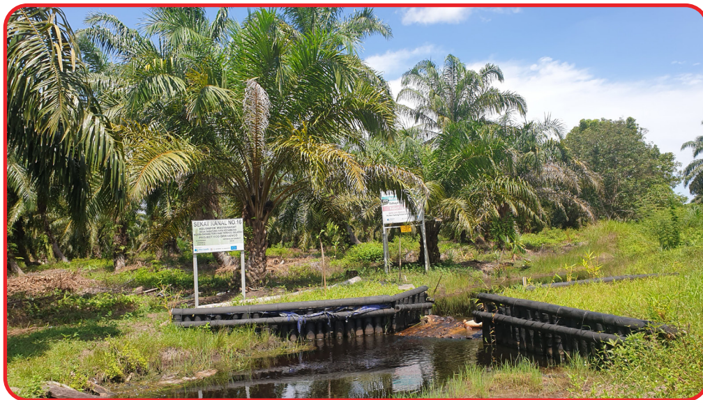
Canal blocking developed by the community groups to effectively keep peatland hydrated. Photo Credit: Malikah Amril/UNEP.
