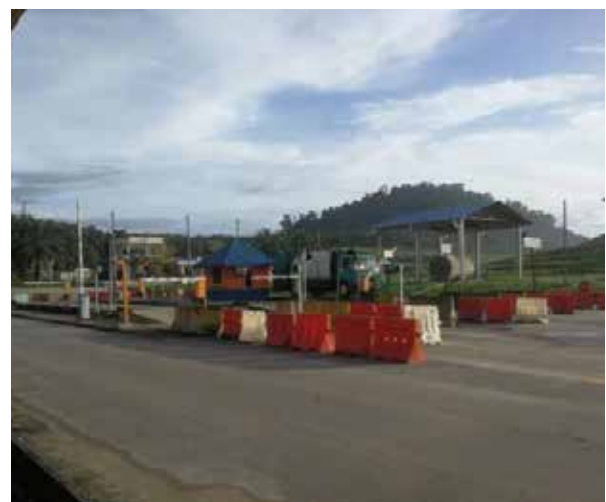
Figure 66: Landfill entrance, weighbridge and active tipping areas
