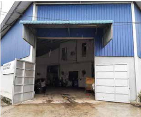
Figure 61: Drop-Off Centre at Bukit Palong for recyclables collected from SAS programme
