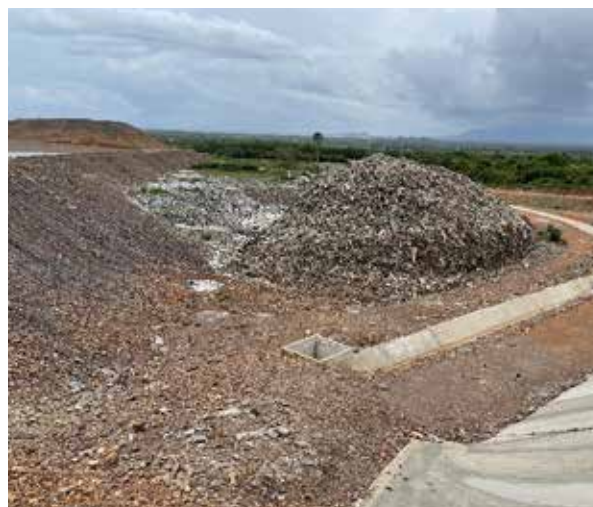
Figure 7: Site visit to the disposal site in Kep City
