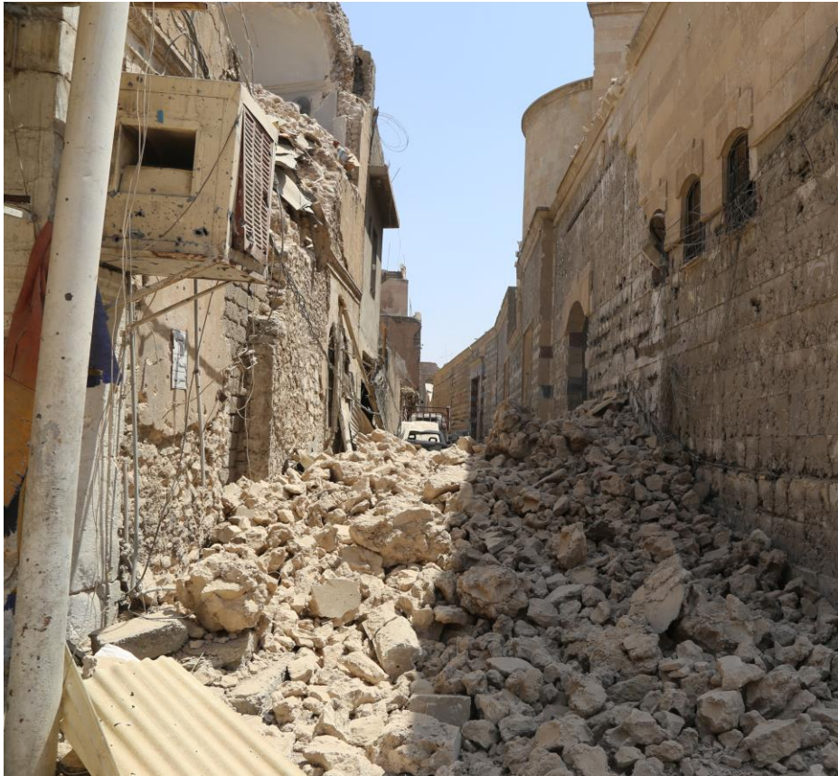
Photos 7 and 8: Small and versatile debris removal vehicles are needed to navigate through the maze-way of Old Mosul's narrow alleyways (typically 1-5 meters' wide)
