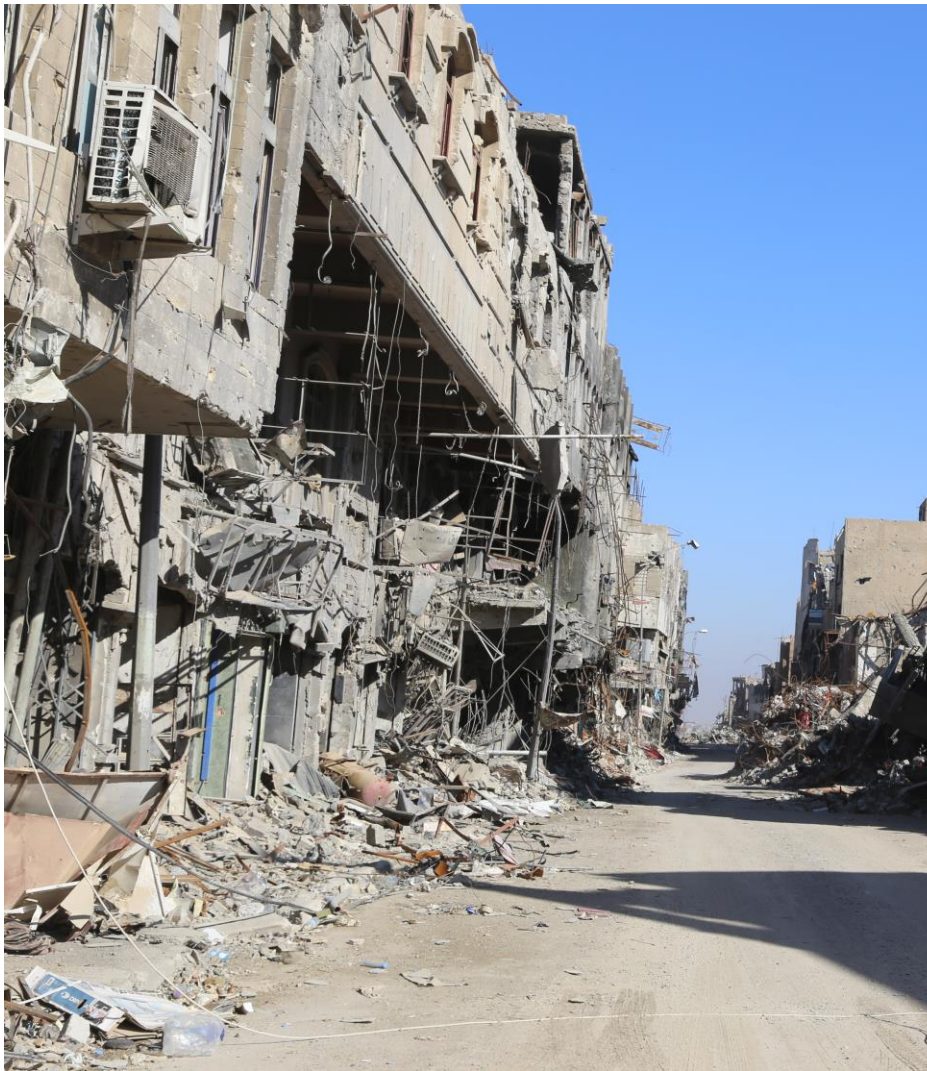
Photo 4: Example of easily accessible rubble on the streets, and 'unreleased' rubble from damaged buildings requiring complex demolition.
