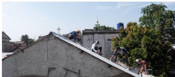
Workers applying a reflective coating to a roof in Tangerang, Indonesia.
