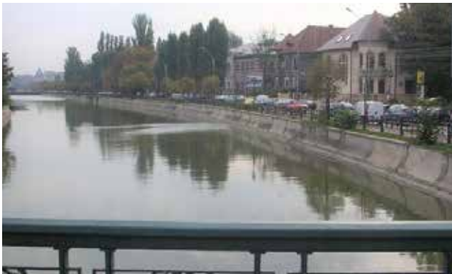
Figure 2.13 Artificial banks along the urban stretch of the Dâmbovița river as it passes through Bucharest © Deborah Chapman
