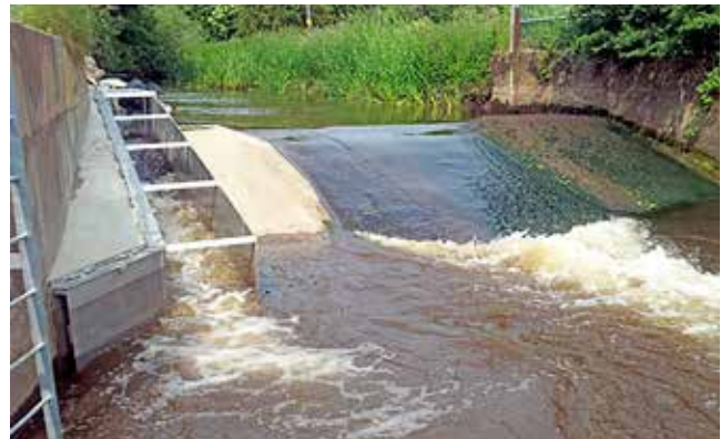
Figure 2.17 The Rodington hydrometric gauging weir on the River Roden with fish and eel pass installed to the left. By Gary Bywater, Environment Agency, UK. Licensed under Open Government Licence v3.0
