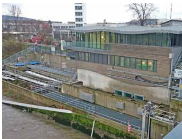
Figure 2.19 Fish pass at the dam on the Moselle River at Koblenz, Germany. The fish are attracted to the outflowing water from the gate at the side of the fish pass © Deborah Chapman
