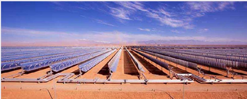
Figure 5.5 Part of the Noor Ouzararte Solar Complex in Morocco
