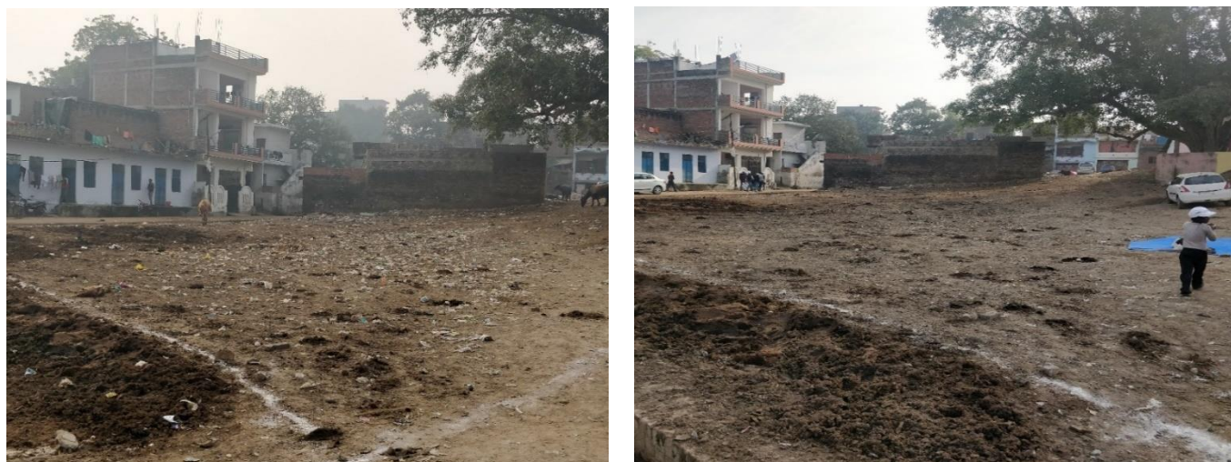
Figure 7: Before and After photographs from the site near Amitabh Bachan Puliya
