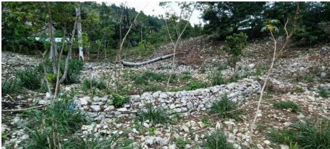
Photo 3: Soil conservation techniques promoted by the project in farms, South Region, Haiti
