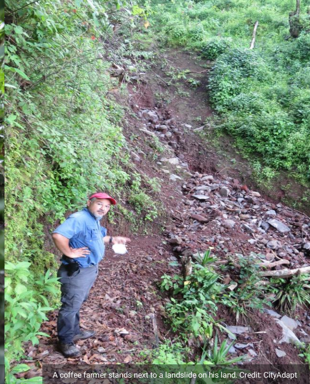
Infiltration ditches were built by the CityAdapt project in coffee farms in San Salvador to reduce flooding. Credit: CityAdapt
