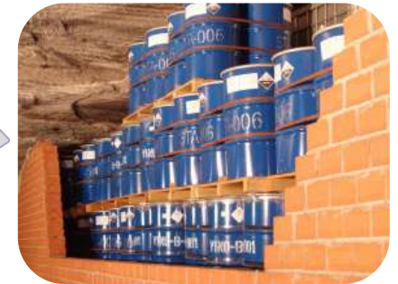
Sealing of by walls
