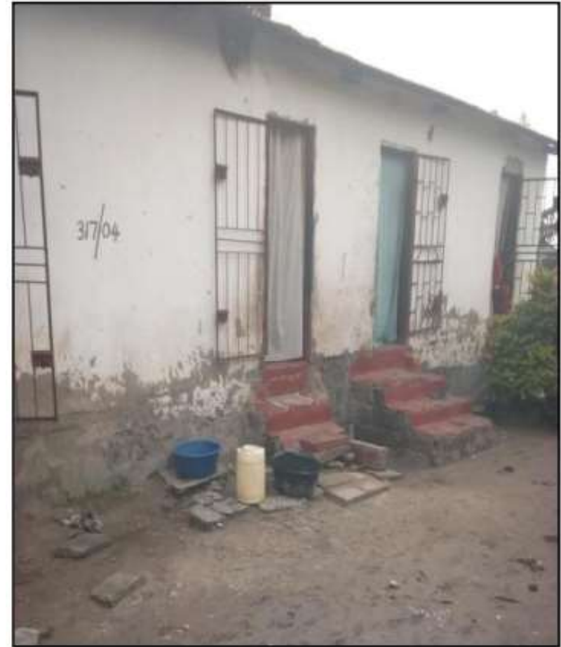
Raised House Foundations
