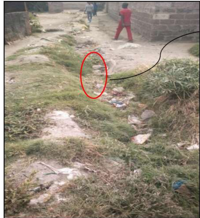
Digging of Small drainages
