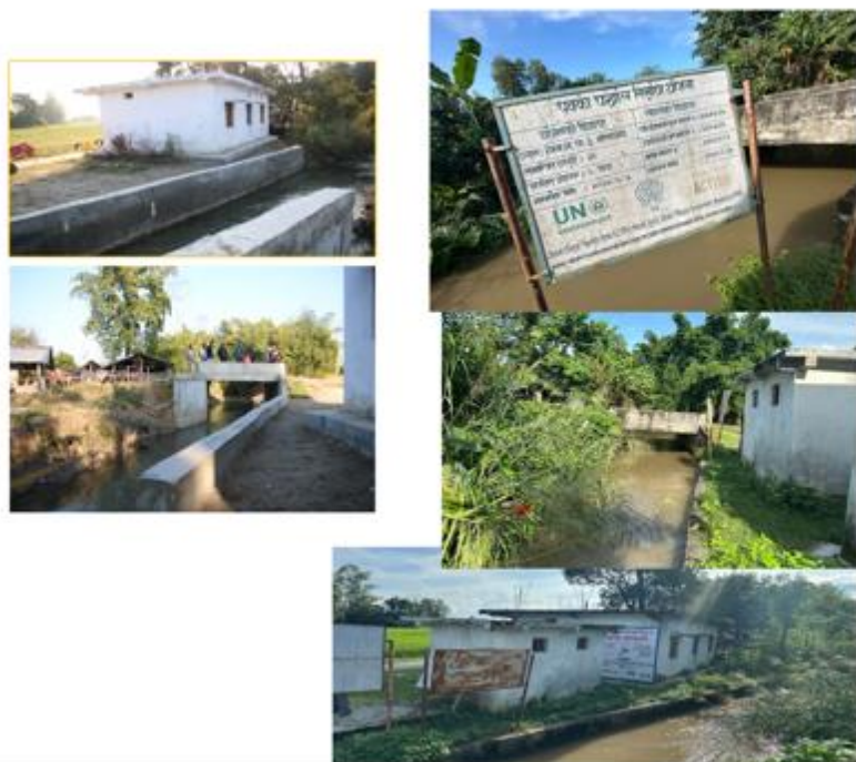
Figure 15 Culvert built at the Tyuni irrigation canal for peacebuilding in Nepal (before and at the time of TE)
