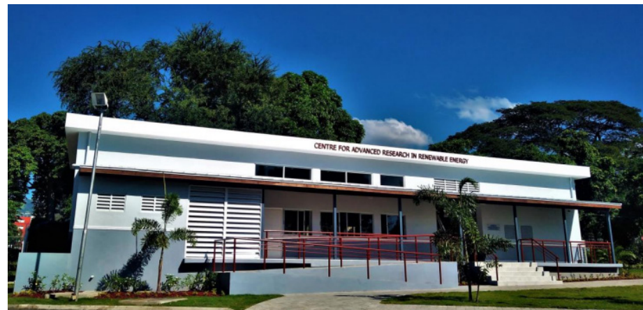
Net-Zero Energy Building, University of the West Indies, Mona, Jamaica. Source: UNEP, 2017.
