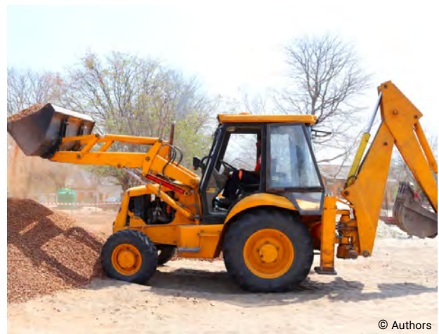
Figure 9: A front-end loader with backhoe
