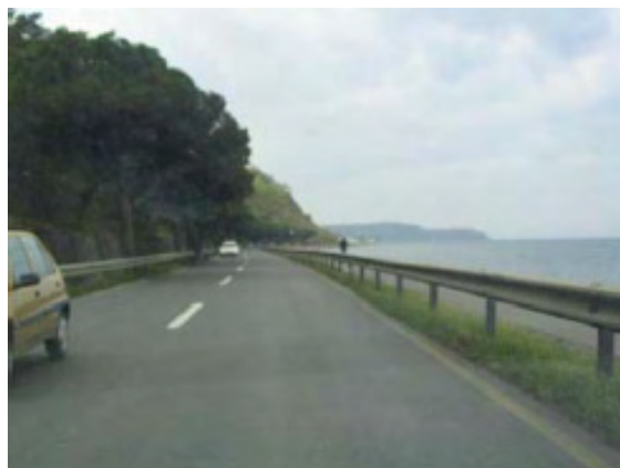
Figure 33: Koper-Izola road occupies an attractive part of the coast below the cliffs
