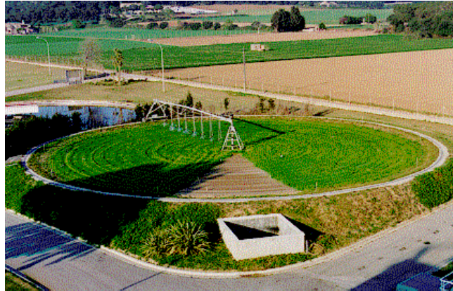
Figure 3.2. Infiltration percolation plant treating secondary effluent in Palamos-Spain
