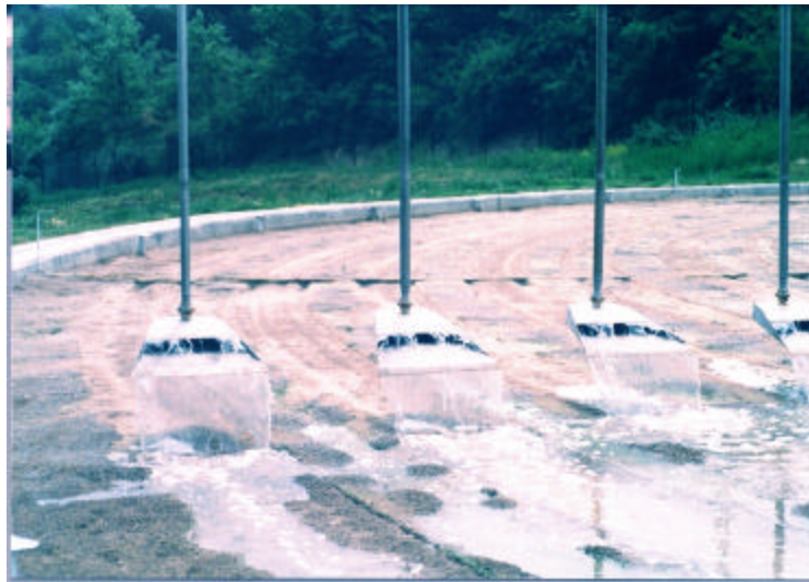
Figure 3.14. Emitters adapted to high SS content effluent.
