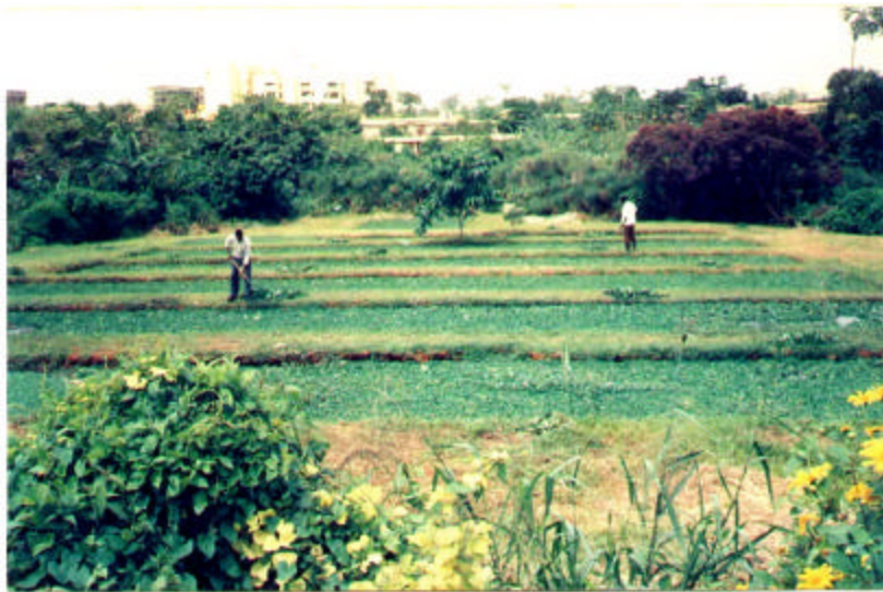
Figure 2.6. Macrophyte-based waste stabilization ponds at Yaoundé (Cameroon)
