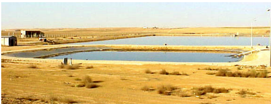
Figure 2.2. Anaerobic pond lined with a plastic membrane at Arad (Israel), with a facultative pond in the background
