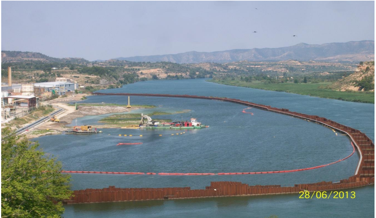
Dredging activities inside the sheet piling
