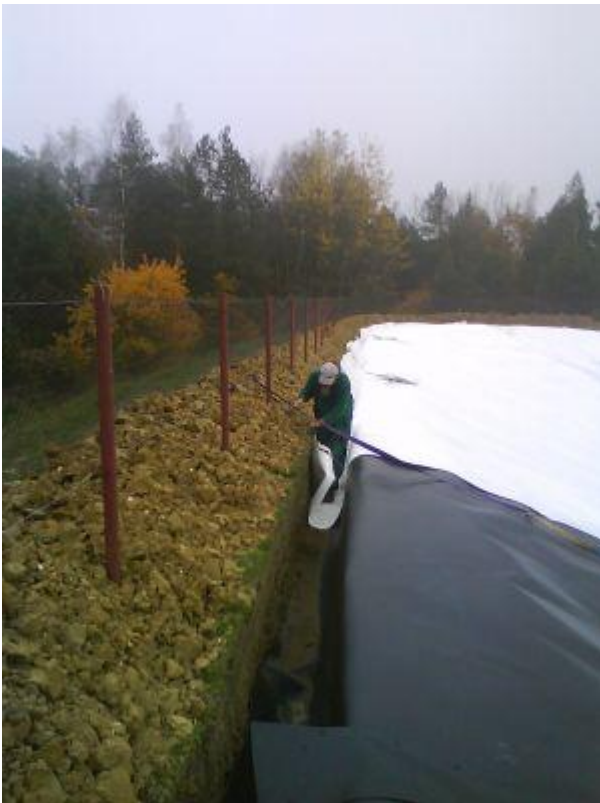
Picture 9: Foundation of landfill
