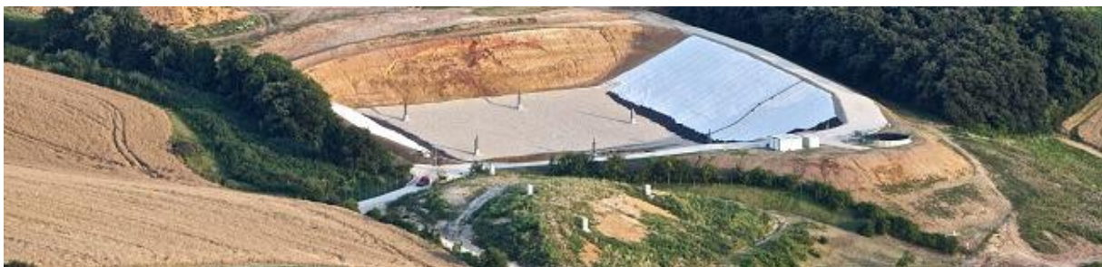
Picture 6: Landfill foundation
