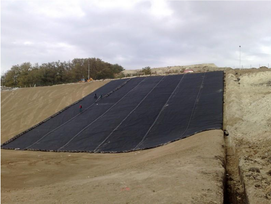
Picture 8: Artificial barrier using HDPE foil for landfill
