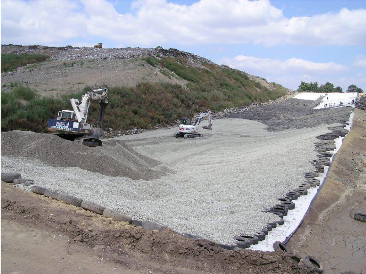
Picture 7: Artificial geological barrier for landfill
