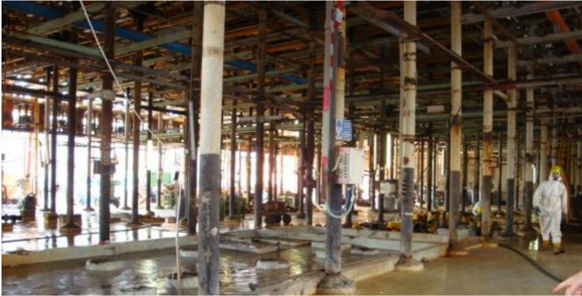
Floor of cell room regularly washed down
