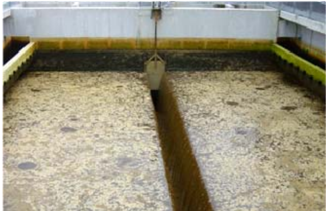
Figure 14. View of backwashing of a high rate gravity sand filter
