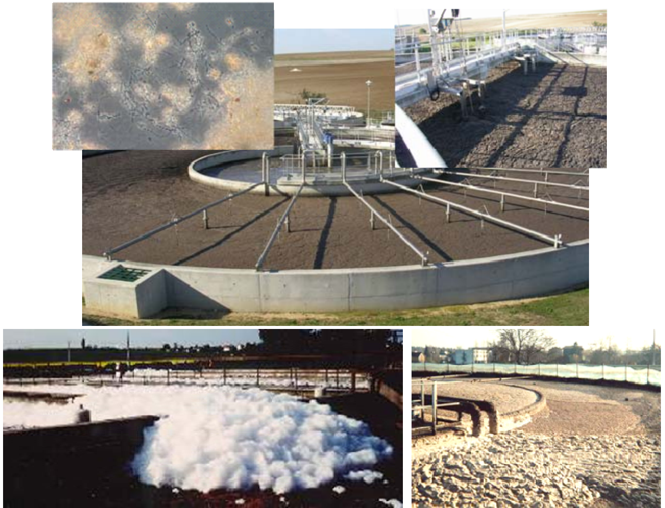
Figure 7. View of foaming in activated sludge systems
