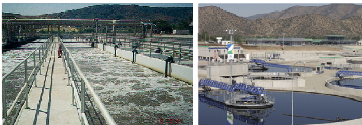
Figure 5. View of aeration tanks and clarifiers
