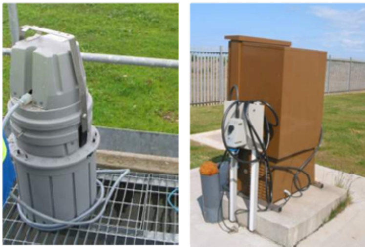
Figure 1. View of a mobile and a fixed automatic wastewater samplers
