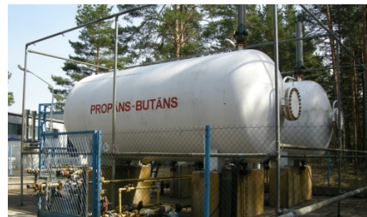
Figure 32: Aerosol manufacturing facility (top) and propane-butane tanks (below). Kvadro Aerosols, Latvia.
