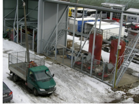
Figure 22: Halon decommissioned from ships using truck and small crane, with storage tanks in background. Halon Bank, Estonia.
