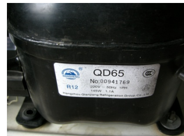
Figure 51: CFC-12 compressor from China. Savodo Teknika, Uzbekistan
