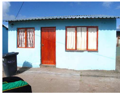
A house in iEEECO Village, with insulated ceiling and fireproof curtains.
