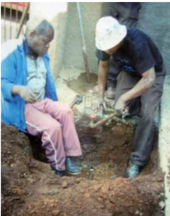
Illustration 55: Measure for fixing the leaks. Retrofitting and exchange of containers (top) and of leaking pipelines on properties (bottom).
