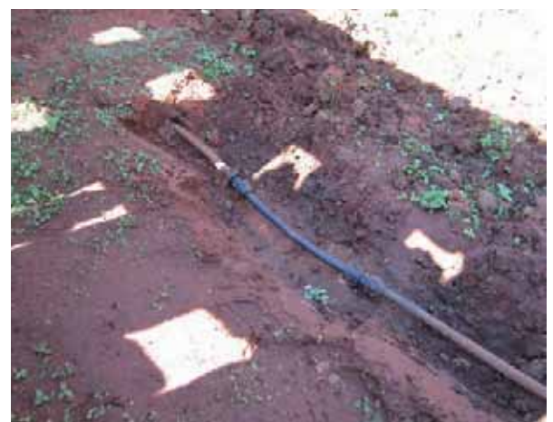
Illustration 55: Measure for fixing the leaks. Retrofitting and exchange of containers (top) and of leaking pipelines on properties (bottom).
