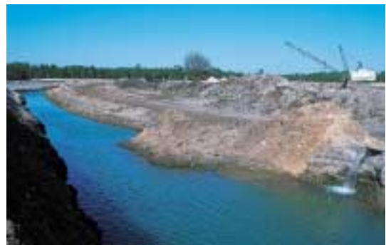
Perimeter ditch - IMC Phosphate, USA
