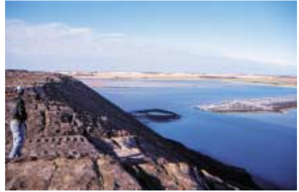
Pond receiving slimes and brine from the stack - Potash Corporation of Saskatchewan (PCS), Canada
