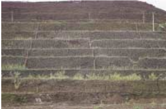
Final pit wall with drains - Copebras S.A., Brazil
