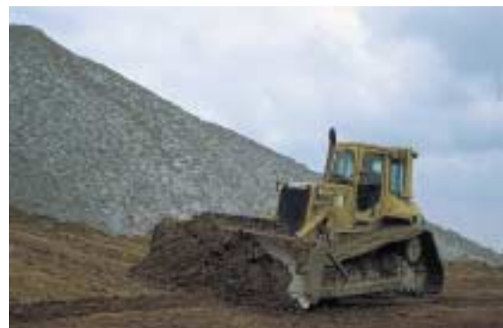
Placing rubble against salt pile - Kali und Salz GmbH, Germany
