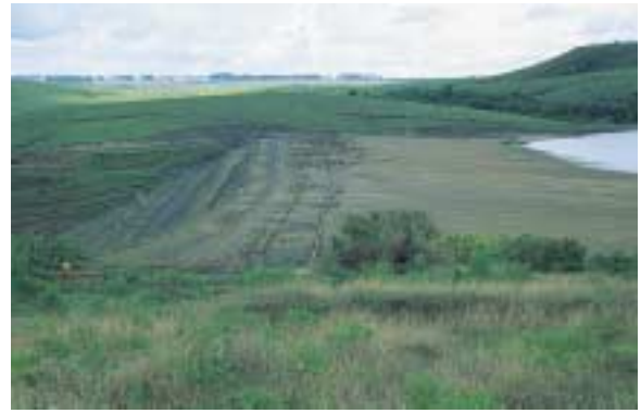
Magnetite tailings dam - Fosfertil, Brazil
