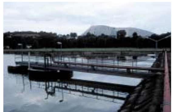
Brine retention ponds for controlled release to Werra River - Kali und Salz GmbH, Germany
