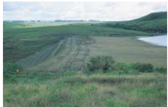
Magnetite tailings dam - Fosfertil, Brazil
