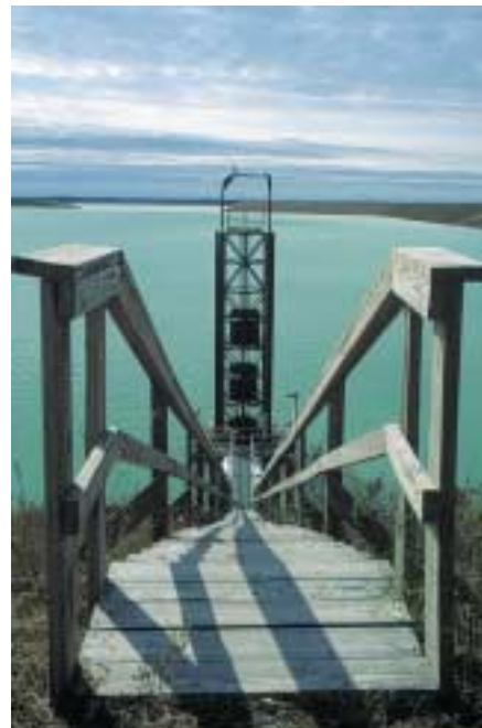
Decantation of clarified water - Cargill Fertilizers Inc., USA
