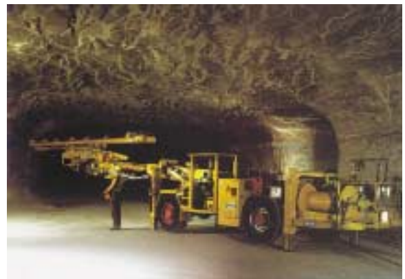
Drilling holes for blasting explosive - Kali und Salz GmbH, Germany
