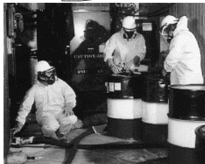
Draining PCBs from an old transformer
