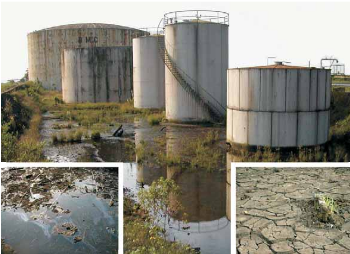
Fuel storage problems in Free Port harbour, Monrovia. Background photo: leaking oil storage tanks. Left: spilled oil in liquid state. Right: oil saturated soil
