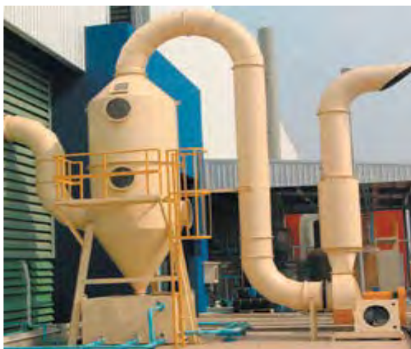
Picture 2.16.1.5.4: A typical scrubber
