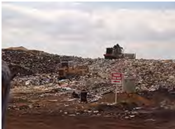
Landfill site in Western Australia
