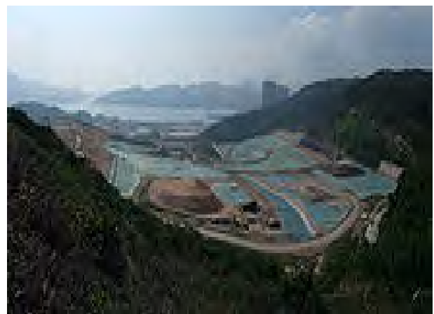
South East New Territories Landfill, Hong Kong
