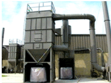
Picture 2.16.1.5.2 A typical cyclone separator
