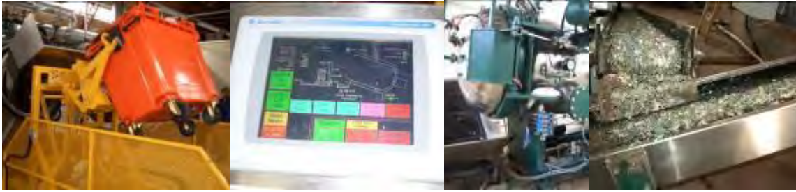
Figure 11.24. (L-R) Automatic bin dumper (L), control panel, Tempico Rotoclave and close-up of treated/shredded waste (R) at the Lautus Central Treatment Plant, Latvia
