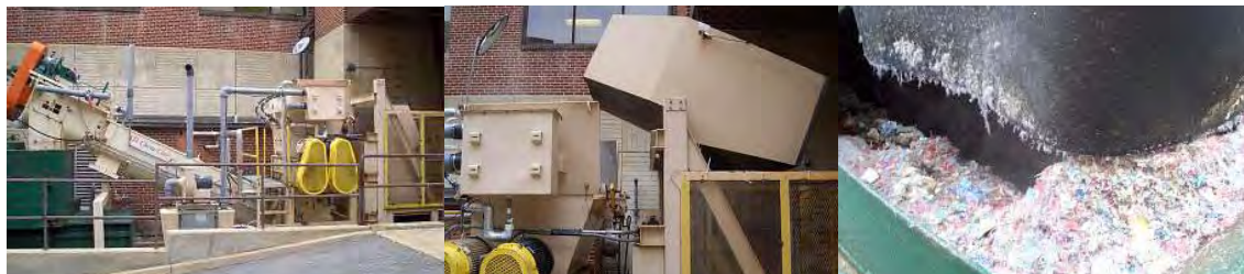
Figure 11.23. STI ChemClav (L), automatic waste dumper (M), and close-up of treated/shredded waste (R) at the Virginia Hospital Center, USA
