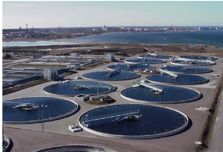
Figure 15- Modern wastewater treatment plant
