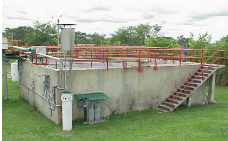
Fig. 2A high rate anaerobic reactor of the UASB type for 6000 population equivalents (research station, Ginebra, Colombia).
