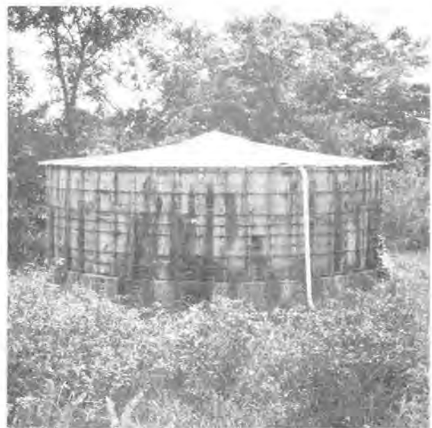
Niue's domestic water is pumped from the groundwater lens into storage tanks before being reticulated to the villages.
