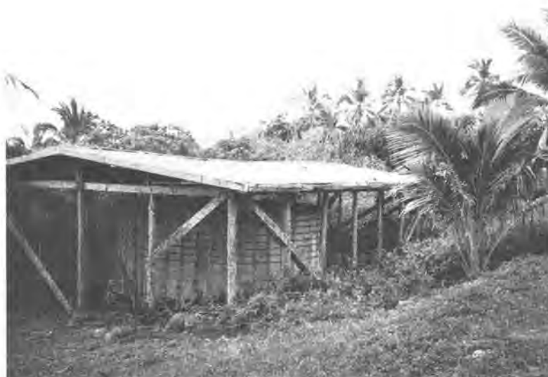
Collecting rainwater in these community catchment systems was common in Niue. Reliance on groundwater, which is piped to individual houses, has led to this older system being mostly abandoned.
