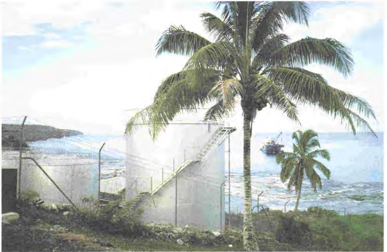
The bulk fuel store at Alofi is not only vulnerable to cyclones but its position means that any accidents lead to a high likelihood of petroleum being spilt into the sea.
