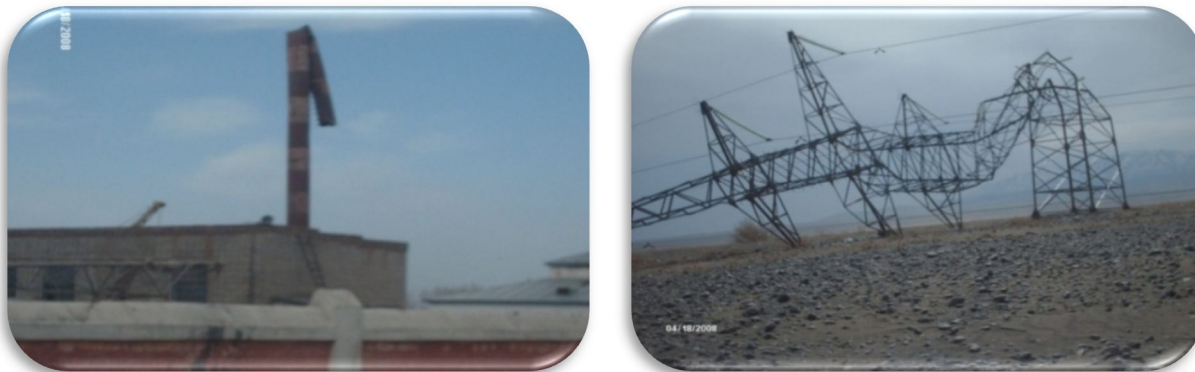
Figure 3. Damages from the strong wind storm of April 18, 2008
