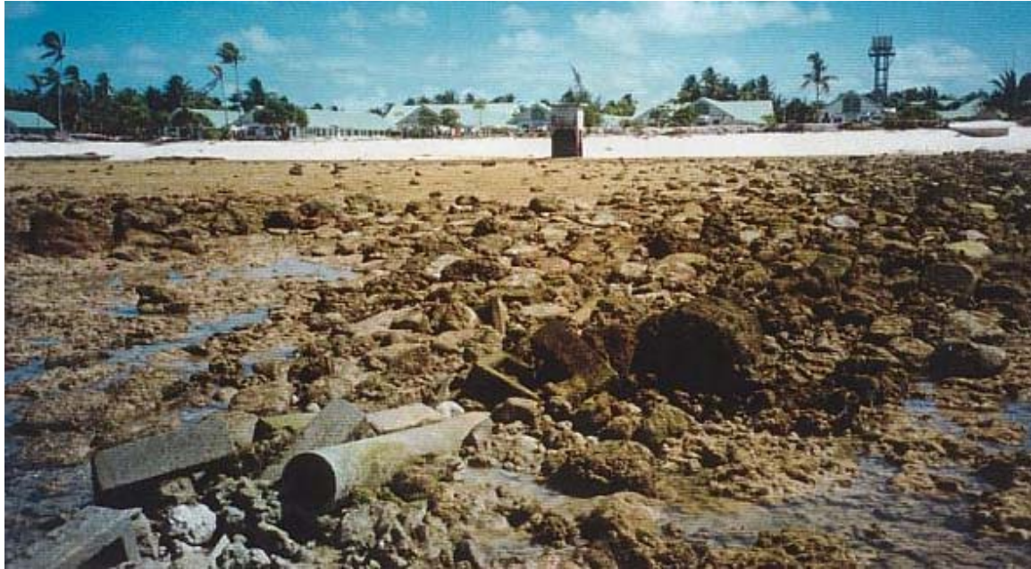
Figure 15.1 Central (Nawerewere) Hospital Outfall at low tide (Royds, 1996)
