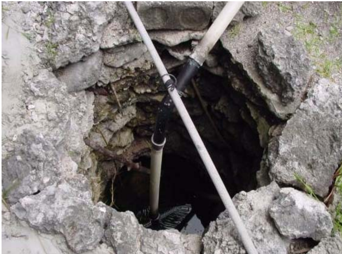
Figure 6. 4 Well water with “Tamana “ pump (ECD, 2000a)
