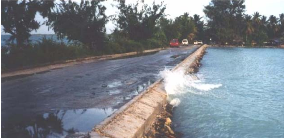
Figure 16.2 Overwash at Steward Causeway, Tarawa (ECD, 2000)
