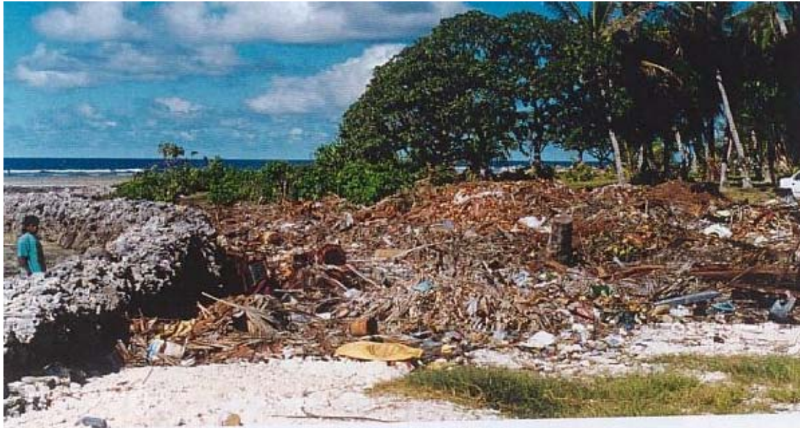
Figure 14.6 Waste tip to be reclaimed with seawall at Teoraeke (Royds, 1996)
