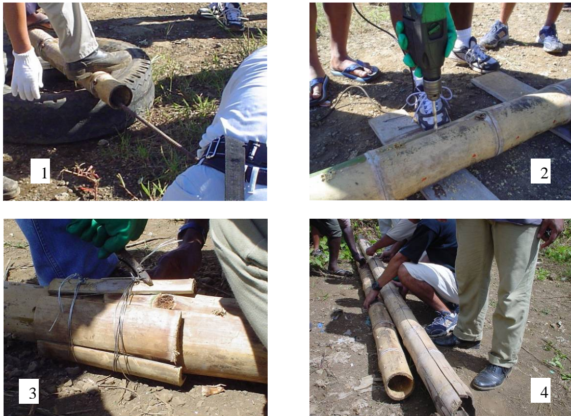
Photo- 18: Bamboos as Substitute Material for Pipes
