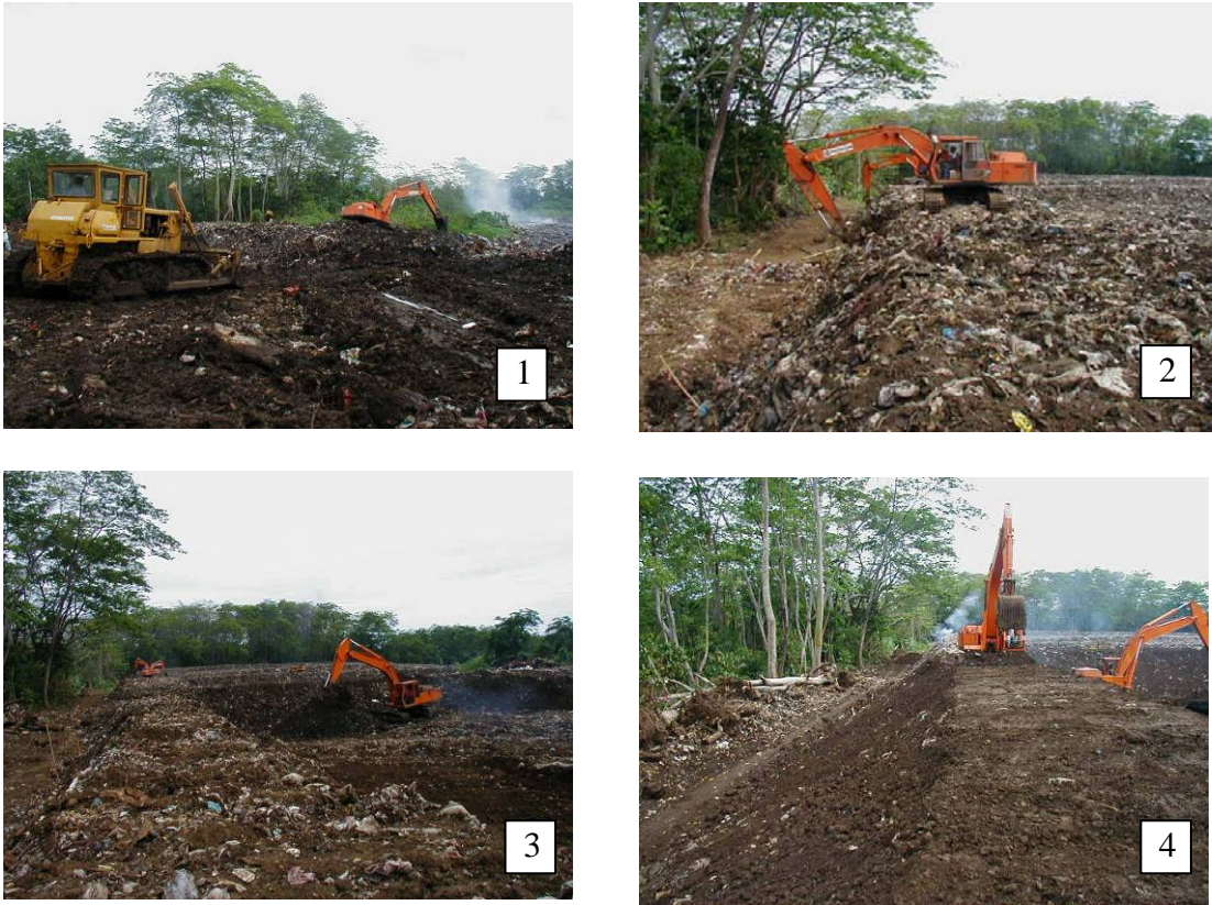
Photo- 16: Sequence of Enclosing Bunds Construction
