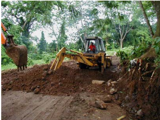
Photo- 14: Excavation of Trench
