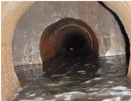
Photo- 43 Clogged Leachate Collection Pipes
