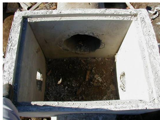
Photo- 24: Pipe Connection Pit
