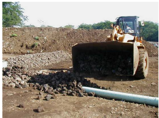
Photo- 20: Installation of Pipes and Protective Gravel Layer
