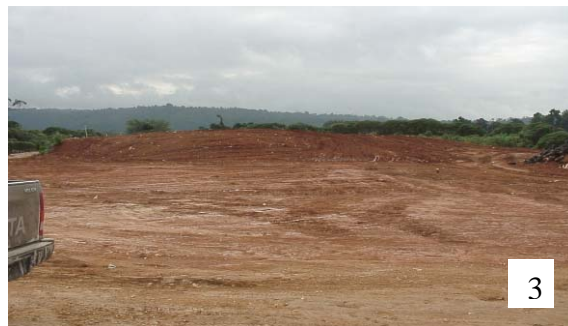
Photo- 5: Transition of Open Dump to Sanitary Landfill (Bouffa Landfill, Vanuatu)
