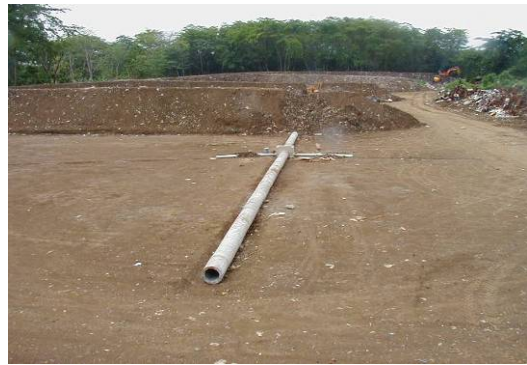
Photo- 19: Concrete Pipe Setting
