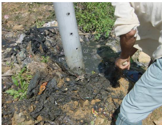
Photo- 44: Clogged Vertical Gas Venting Pipes
