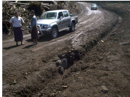
Photo- 12: Side Ditch with Road Crossing Culvert
