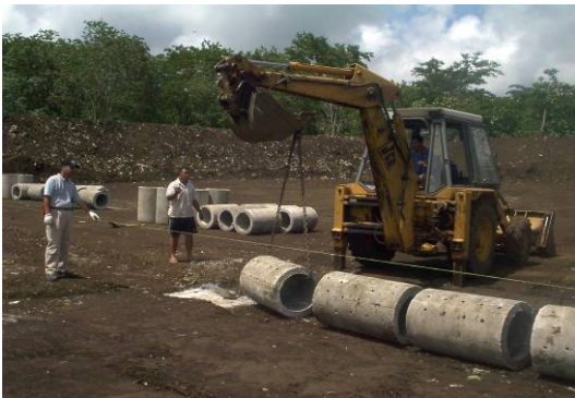
Photo- 19: Concrete Pipe Setting
