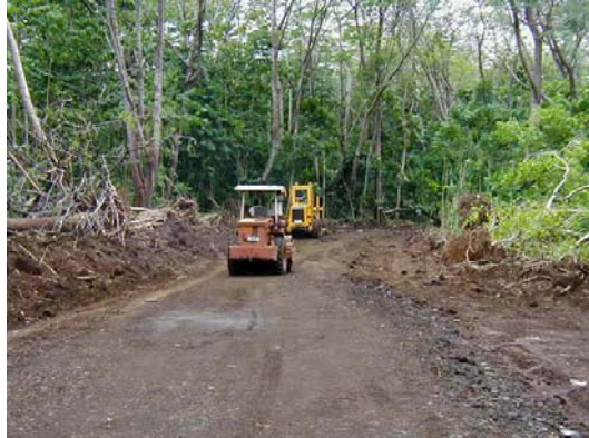
Photo- 9: Compaction & Gravel Paving
