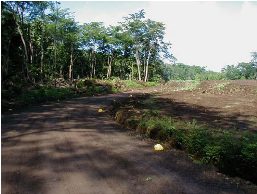
Photo- 11: Side Ditch with Curb Stone
