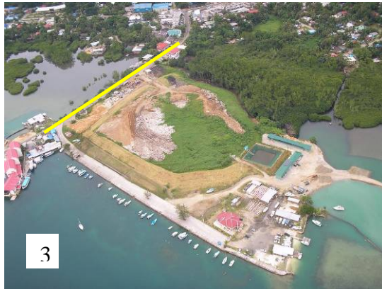
Photo- 4: Transition of Open Dump to Sanitary Landfill (M-dock Landfill, Palau)
