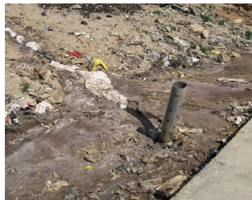
Photo- 44: Clogged Vertical Gas Venting Pipes
