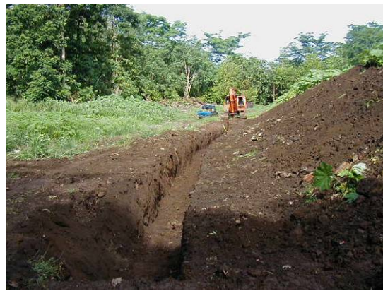
Photo- 13: Perimeter Drain Excavation
