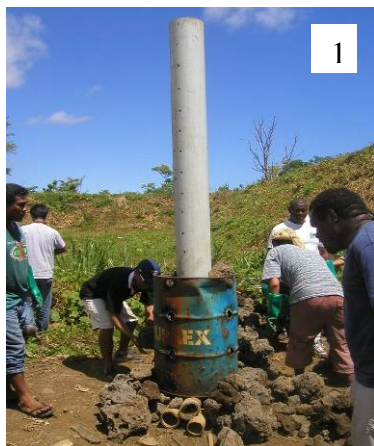
Photo- 27: Vertical Gas Venting Pipes at Landfilled Area
