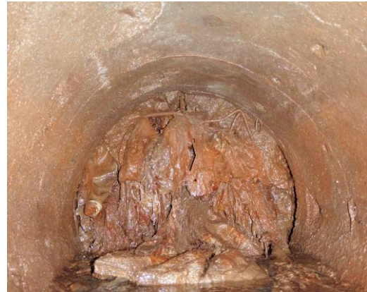
Photo- 43 Clogged Leachate Collection Pipes
