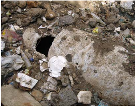
Photo- 42: Damaged Leachate Collection Pipes
