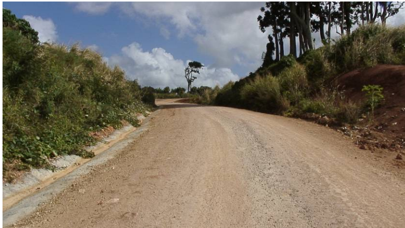
Photo- 40: Example of Site Access Road (Bouffa Landfill, Vanuatu)
