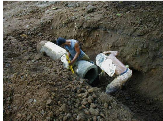
Photo- 15: Diversion Pipe Setting
