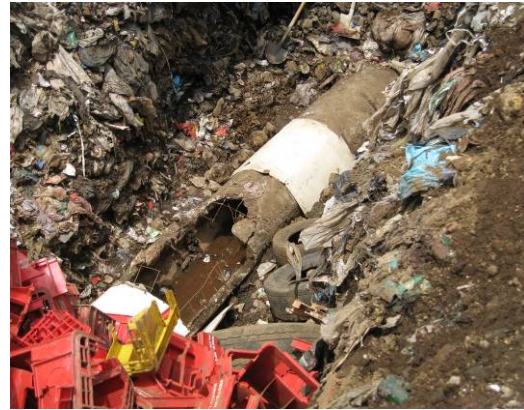
Photo- 42: Damaged Leachate Collection Pipes
