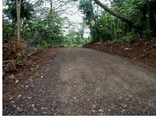
Photo- 10: Paved Access Road
