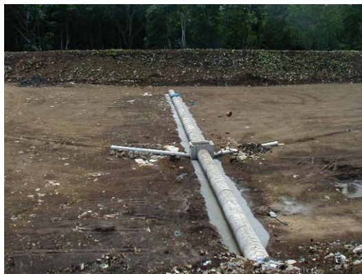
Photo- 20: Installation of Pipes and Protective Gravel Layer
