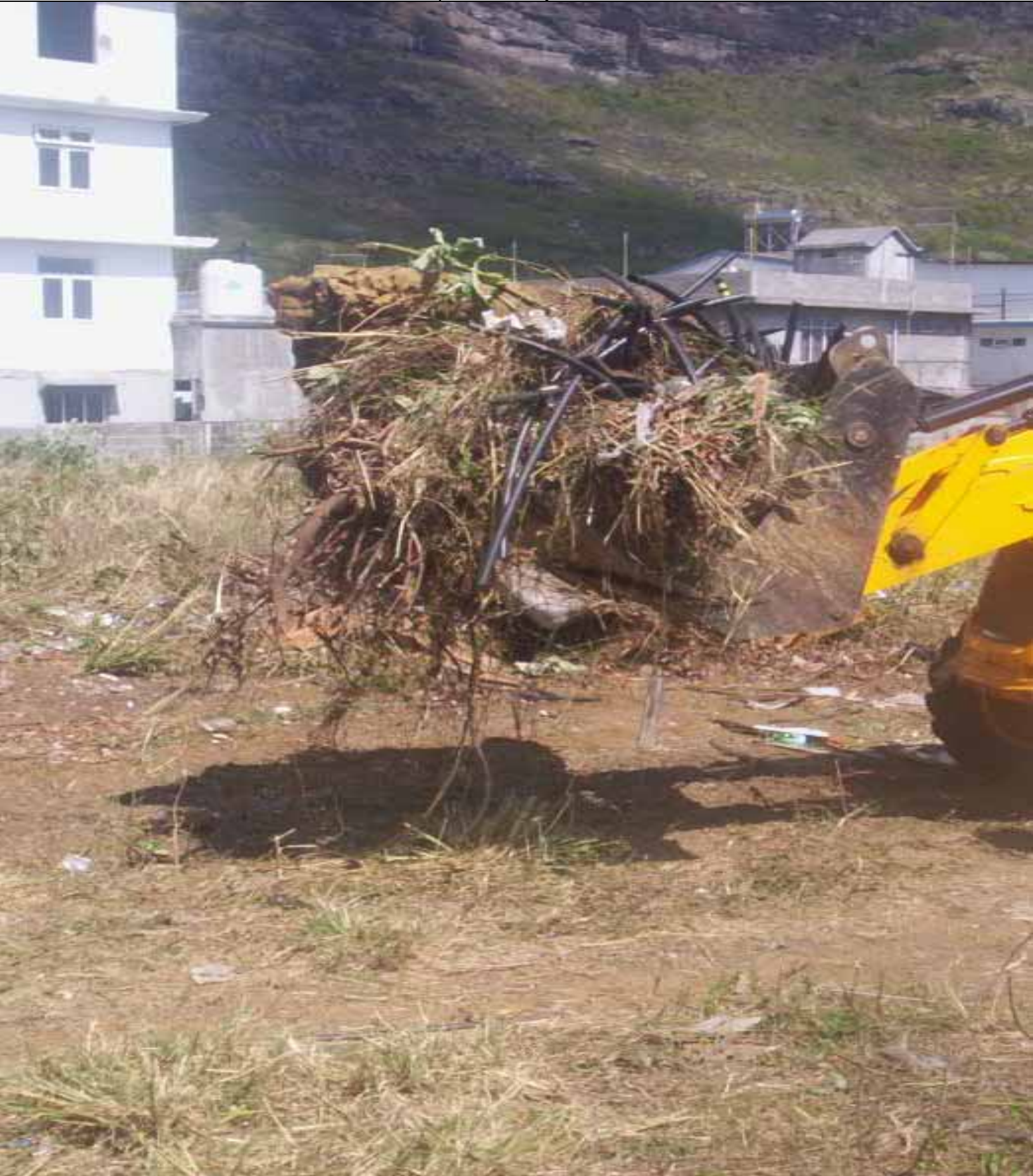
Before Clean Up at Boundary Road, Quatre-Bornes
