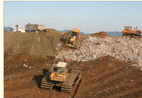
● Soil Covering Process during Sanitary Landfill
