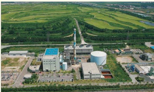
● View of Landfill Site 1 where Dream Park Golf Course will be constructed, and 50MW Landfill Gas Power Plant
