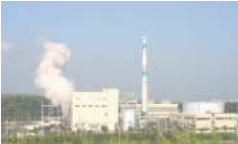
< The 50MW Power Plant >
