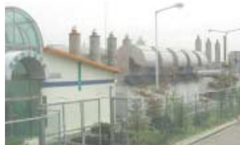
< 9.88MW Power Plant >
