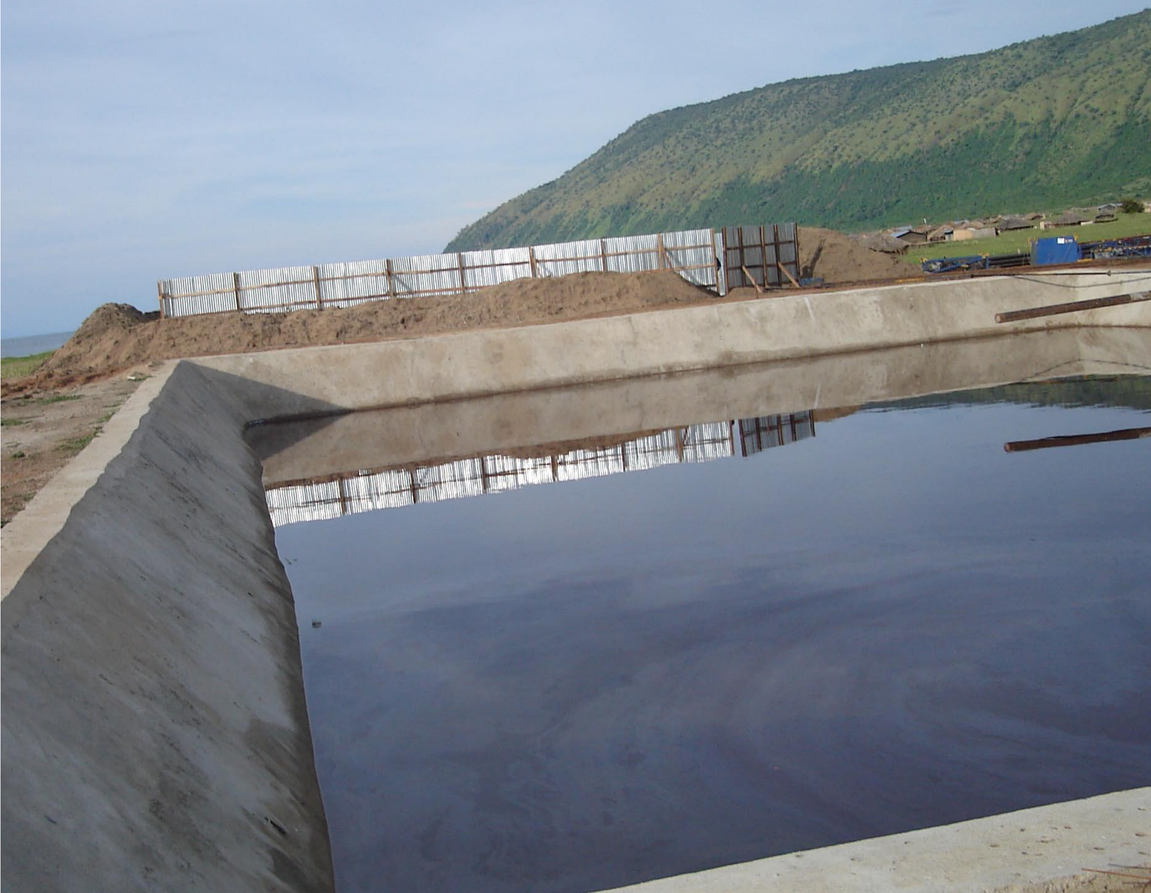
Fig. 2: A concrete lined waste mud and cuttings pit at Kingfisher in Bugoma, EA 3A. Source: Petroleum Exploration and Production Department (PEPD) 2006
