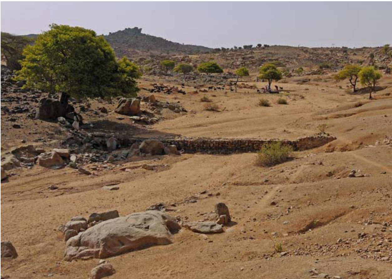
A sand dam and well in the Red Sea Hills. Maintenance in this catchment management project relies on collaboration of the communities in the valley who contribute labour and money to safeguard water resources and reduce soil erosion
